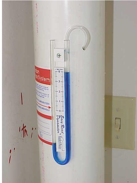
Picture 18. Interior-mounted U-tube.
