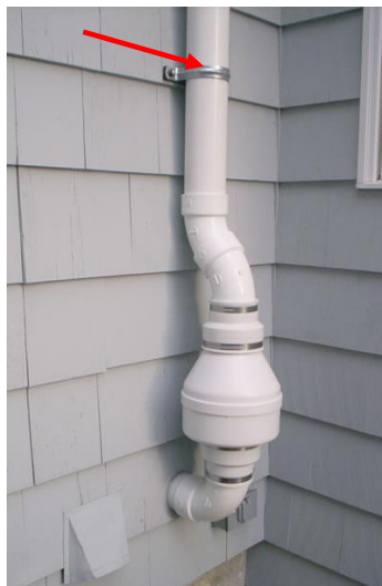
Picture 15. Wall-mounted friction-based pipe strap (not recommended).
