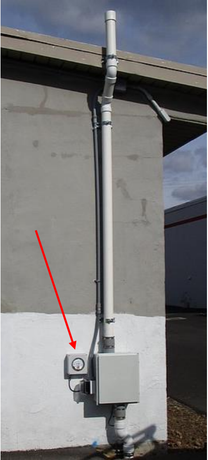
Picture 20. Magnehelic performance indicator.
