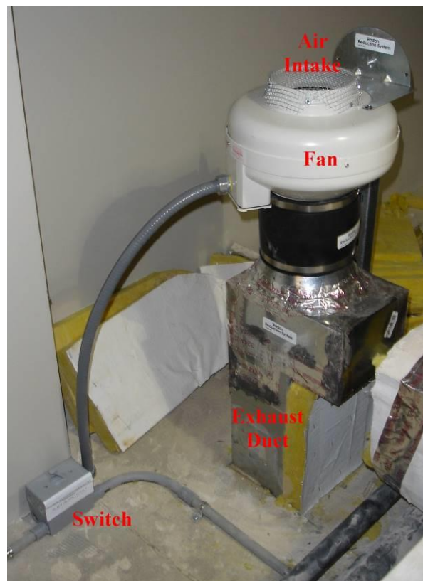
Picture 34. SAM components with centrifugal fan.
