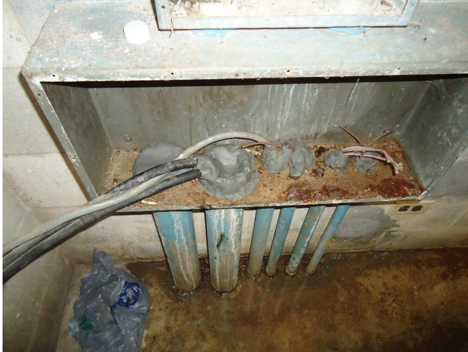
Picture 23. Passive sealing of a radon entry pathway
