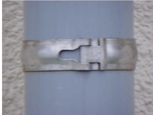
Picture 14. Clip on friction-based pipe strap (not recommended).
