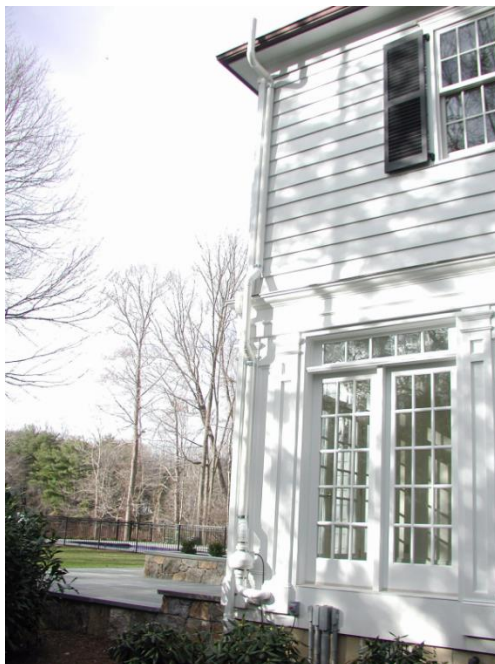
Picture 12. Properly vented SSD mitigation system.
